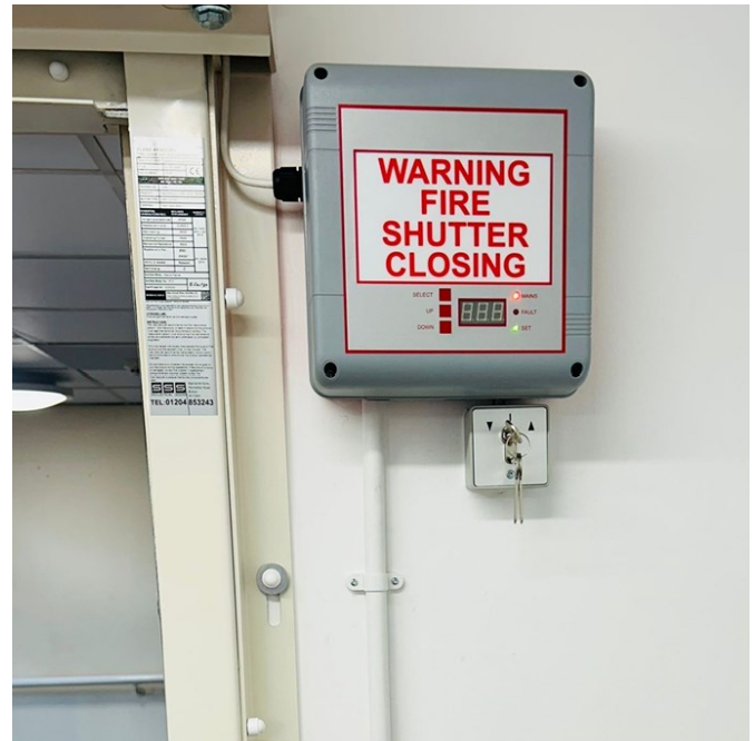
EXAMPLE OF CABLE ROUTING ON A FLAME ARMOUR+ FIRE RESISTANT ROLLER SHUTTER
